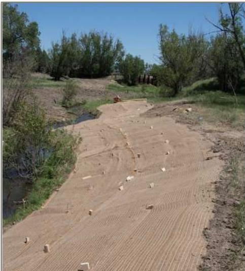
After the bank slopes are fine tuned, we use a seed drill plant native seed. Then we use coconut mats to hold the soil as shown here. Erosion control mats like this help keep the soil in place, helps to retain moisture in the soil, and lets sunlight through to allow those seeds to germinate and have the best start.
